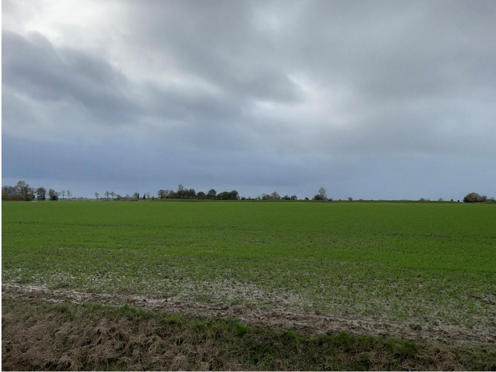
Figure 106. Remnant of dike structure (Ooster-Waarddijk) in the distance
