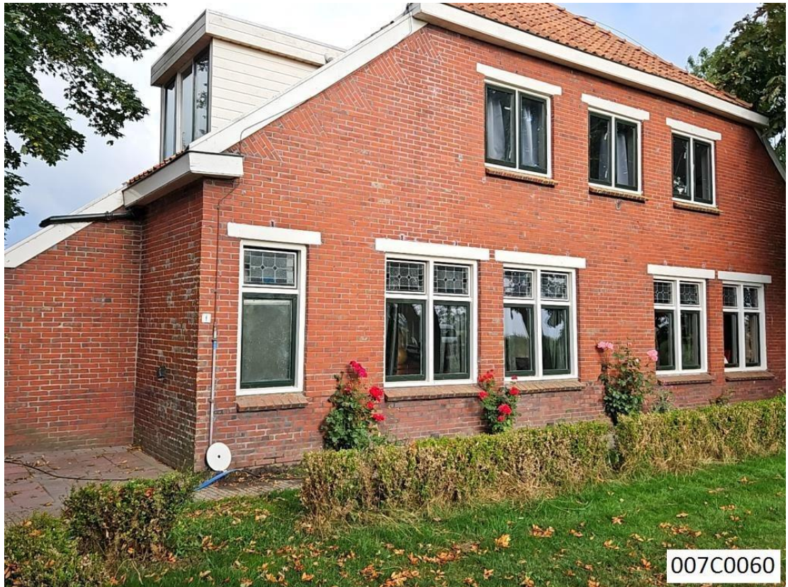
Figure 1. A house with a benchmark which is highlighted for the purpose of this photo using a white disk around the benchmark. (Source: NAP Info)
