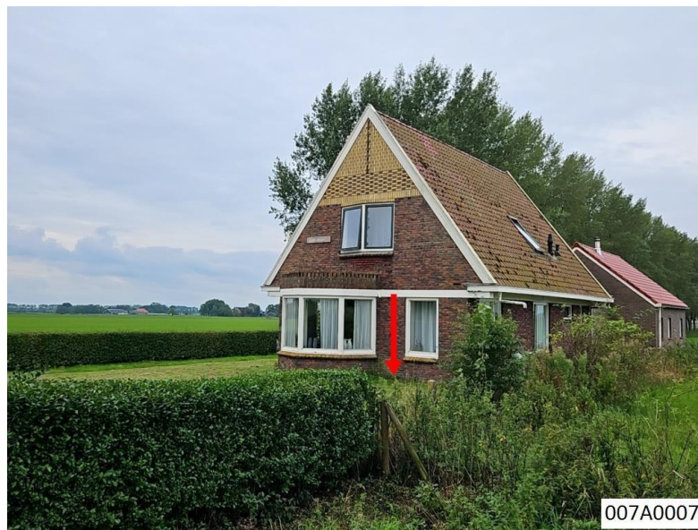
Figure 88. Location of point 007A0007, indicated by a red arrow.
